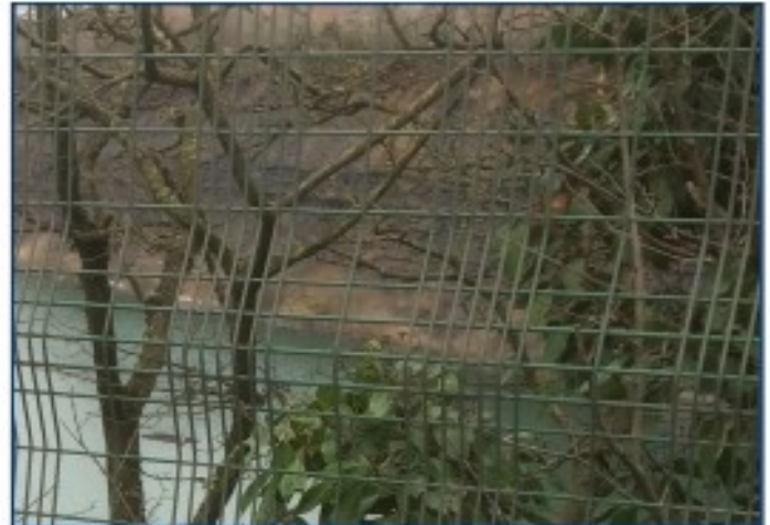
Parkfield Road quarry work is underway
